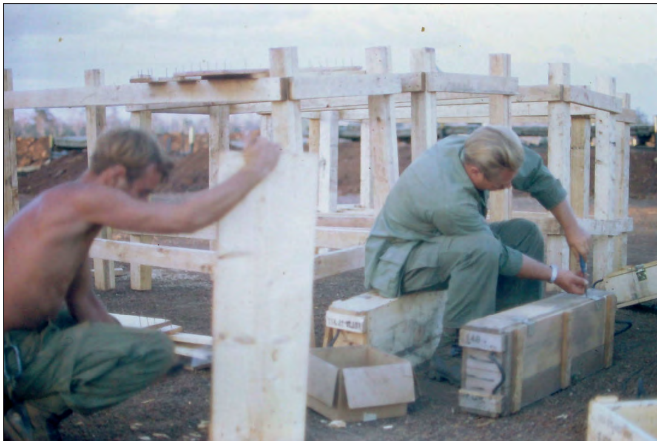
Building bunks from wood salvaged from 105mm ammunition crates. The soldier on the right is disassembling one of the crates.
