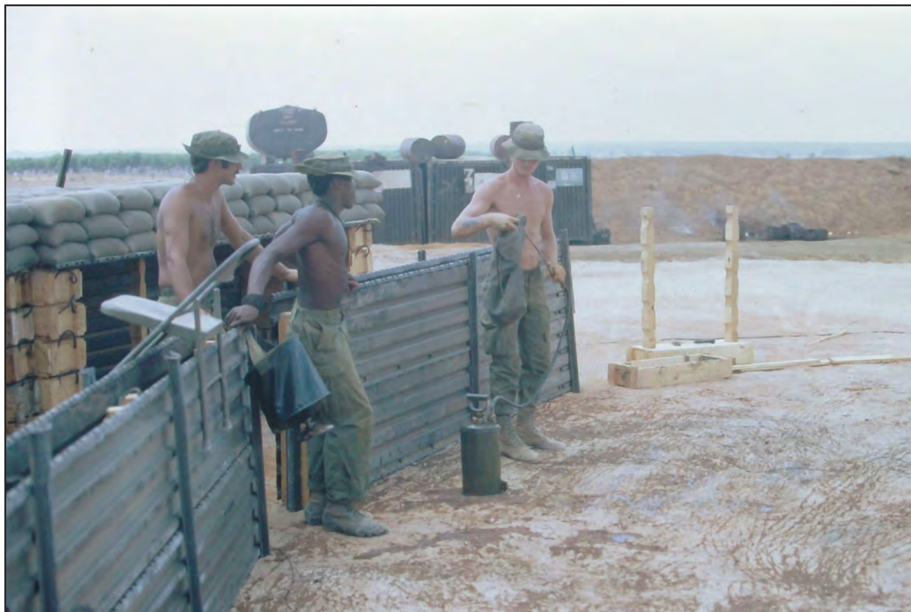
Note the metal rods holding up the metal sheets of the blast walls.
