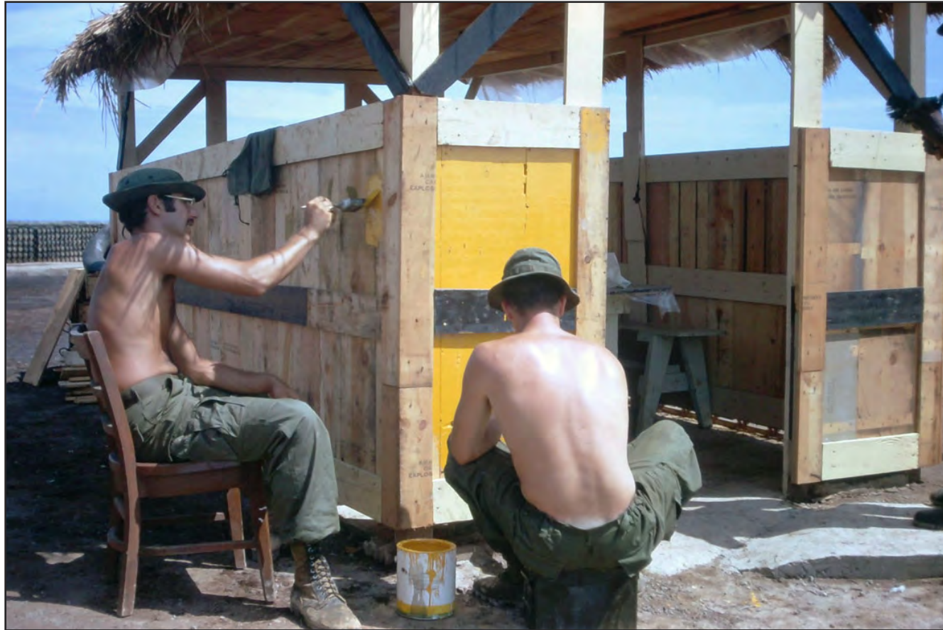
Painting the sides of one of the sheds. This one had wooden sides made from disassembled ammunition boxes.
