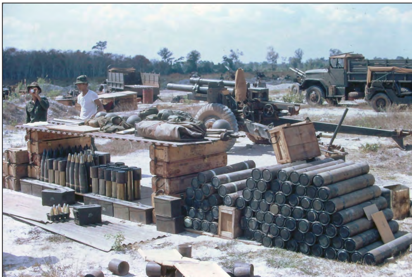
The ammunition bunker for the 105mm howitzers under construction. The wooden boxes are crates used to transport the 105mm ammunition, and when empty served as building blocks for the ammunition bunker. The long dark tubes each held one 105mm howitzer round, including the shell and the powder. The metal cans held fuzes for the shells.
