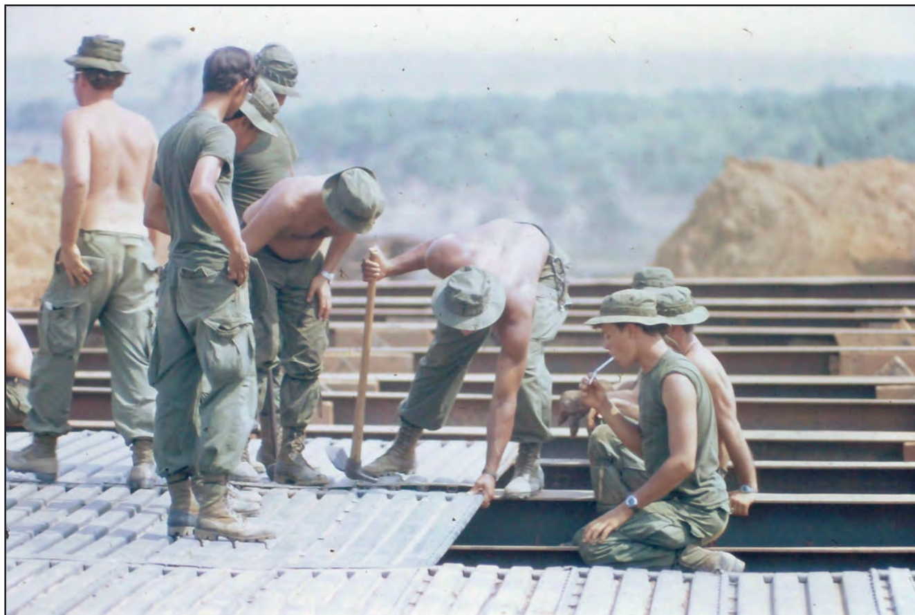
The roof on the ammunition dump was made of interlocked metal sheets usually used for helicopter landing pads. Later this roof would have several layers of sandbags installed for additional protection.
