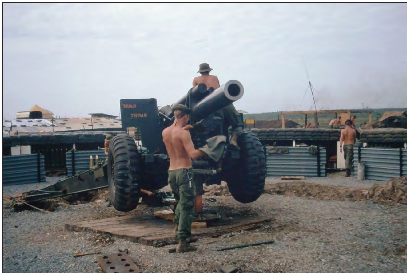
A howitzer emplacement nears completion. Note that gravel has arrived.
