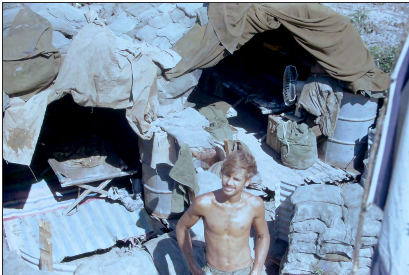
The entrances of two living quarters at Andrews. The roof structure was made of pieces of metal culvert covered by sandbags, and the floors were sheets of metal planks normally used for helicopter landing zones.
