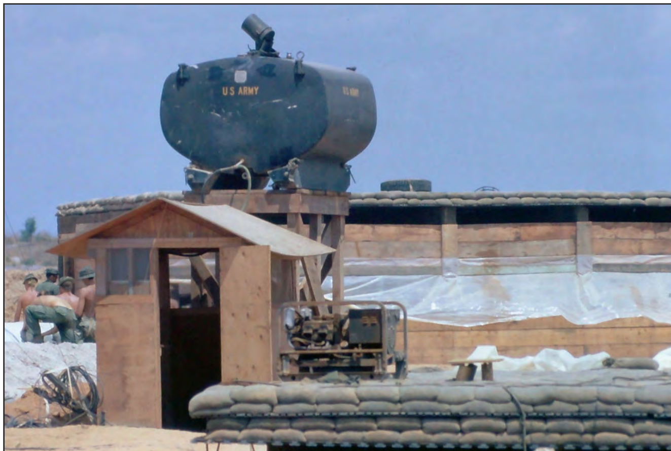
Another water tank mounted on a tower. The mess hall is in the rear, with the serving windows protected by sheets of plastic. Note the two rows of sandbags protecting the top of the mess hall.
