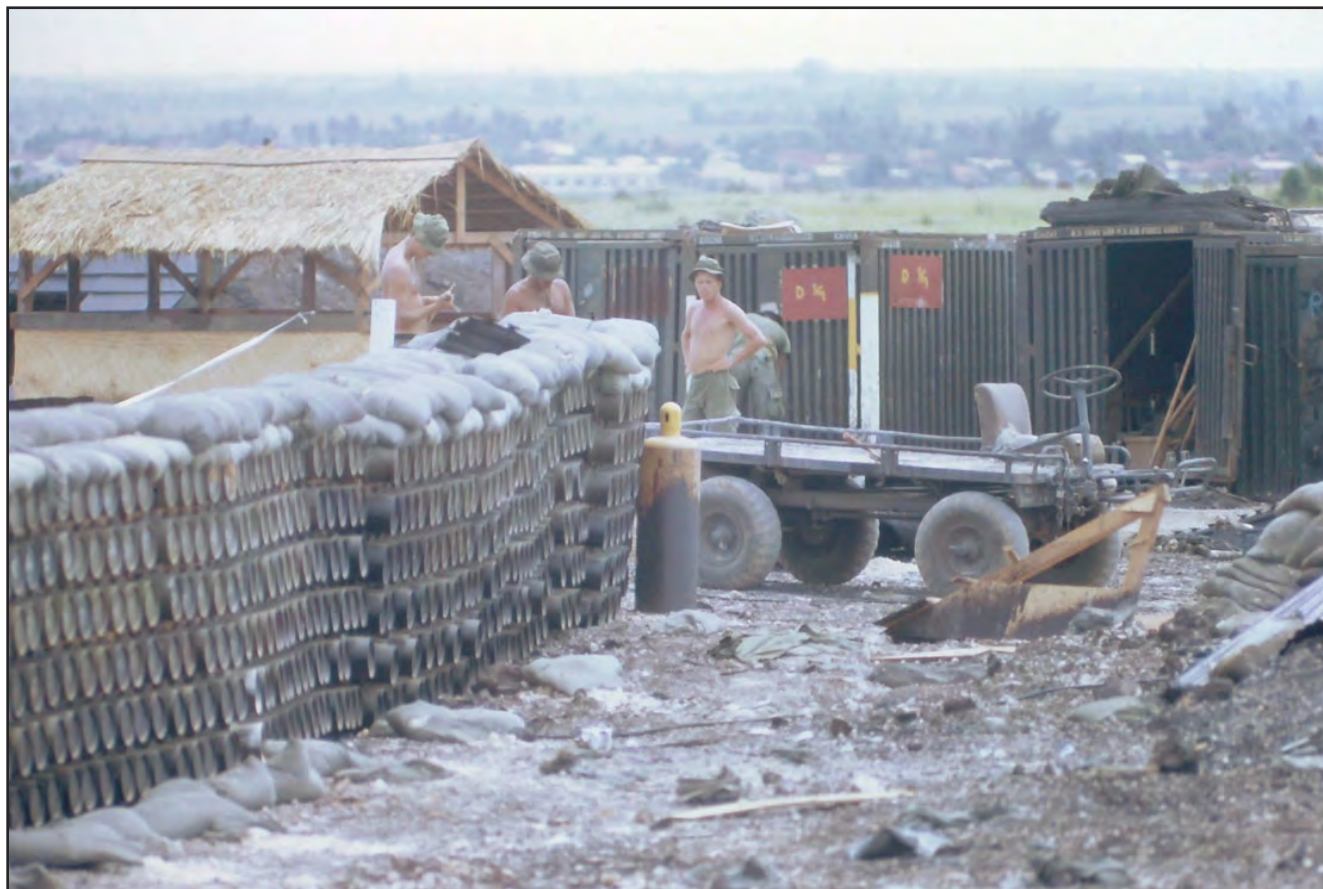
The blast of the explosion damaged the back of the protective wall around one of the howitzer emplacements. The dirt-filled canisters in this wall would normally have been arranged in a perfectly curved line.
