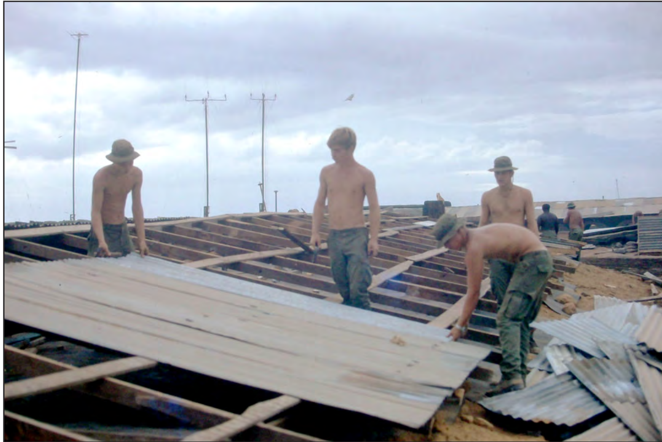
Installing the light metal sheets on top of a roof structure.
