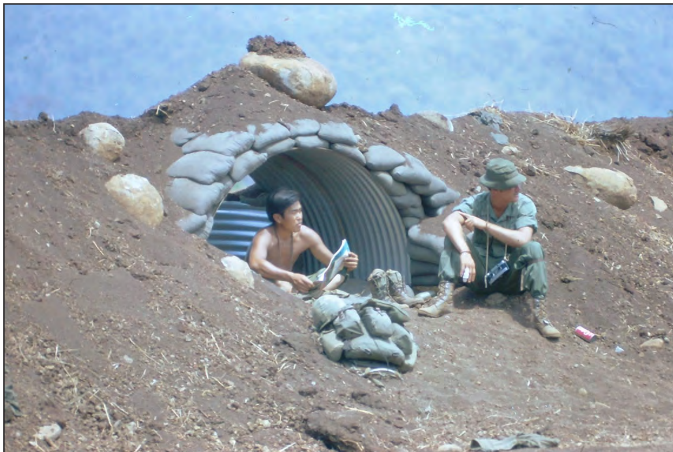
One of the guard posts on the perimeter “berm,” or wall of dirt pushed up to make a protective wall. This guard post was manned every night from dusk to dawn and during daylight hours if security conditions required.
